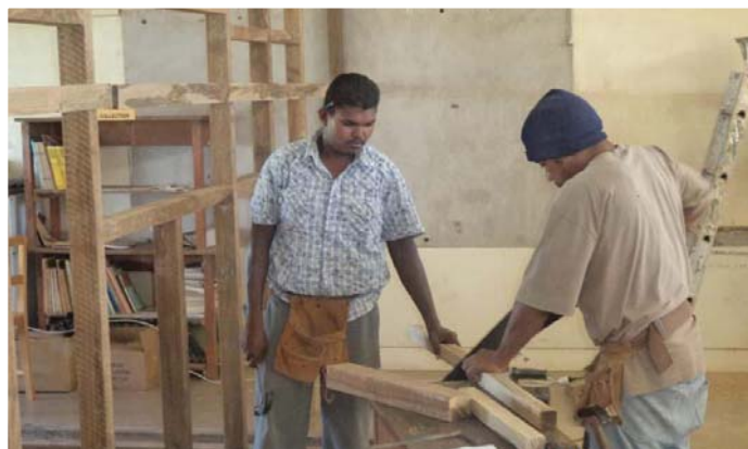
New computer Lab, under construction, will house the ICT equipment
